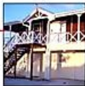
Secondary Voltage Power
