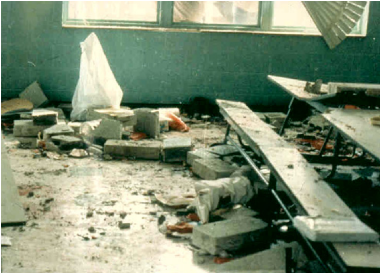
School cafeteria after a hot water tank explosion
